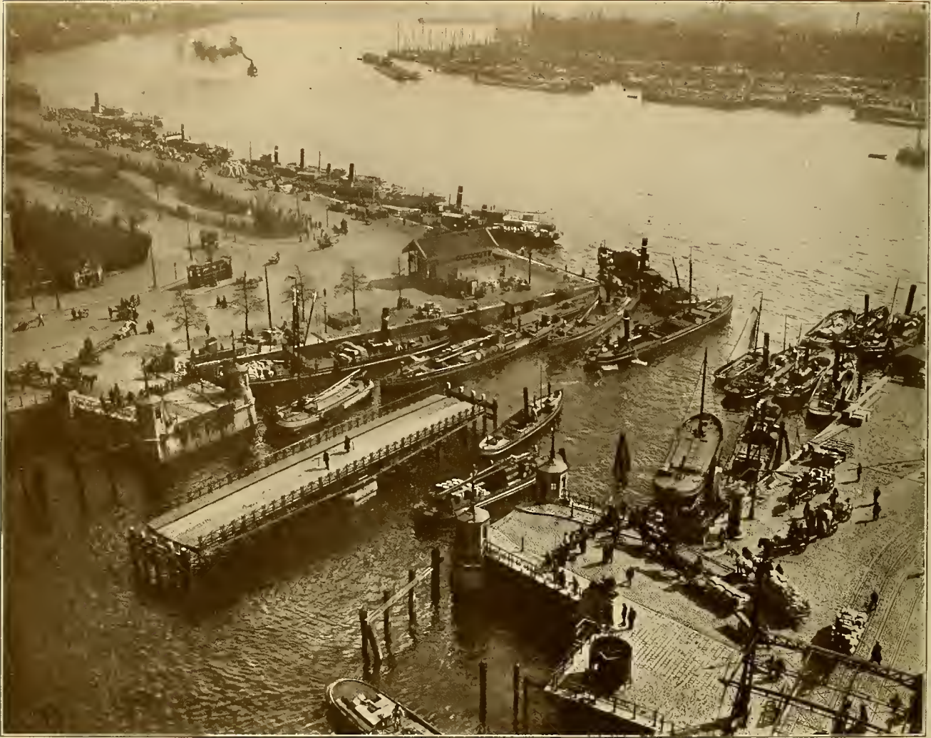
THE "OOSTERKADE", A BUSY RIVER TRAFFIC SECTION AT ROTTERDAM
